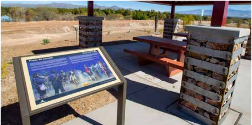
Recently completed trailhead in Marana along the Juan Bautista de Anza Trail.
