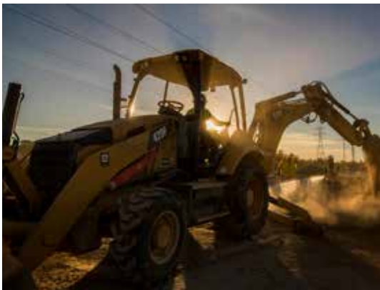
New Pima Animal Care Center under construction.
