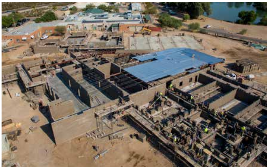
New Pima Animal Care Center under construction.
