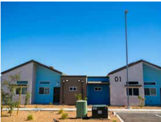
Esperanza en Escalante Veteran Housing, Completed June 2017.
