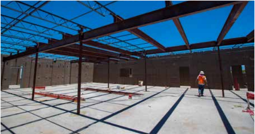
New Pima Animal Care Center under construction.
