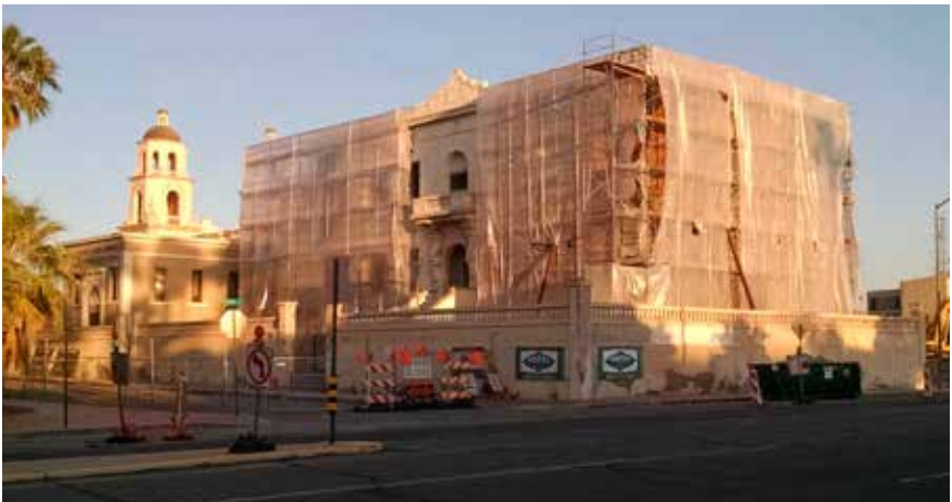
The Marist on Cathedral Square, Senior Rental Housing under construction.
