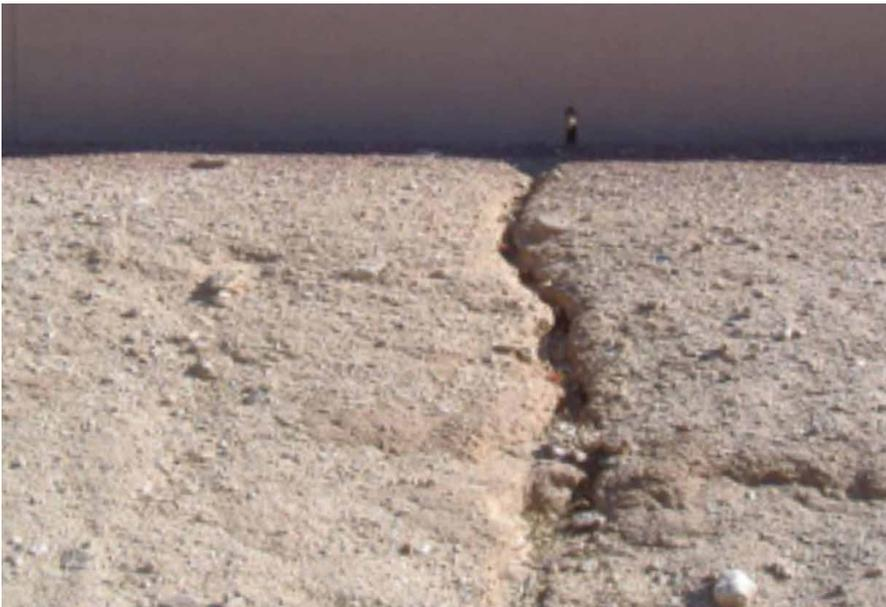
**A wall opening into a basin that has created erosion on the basin slope.**
