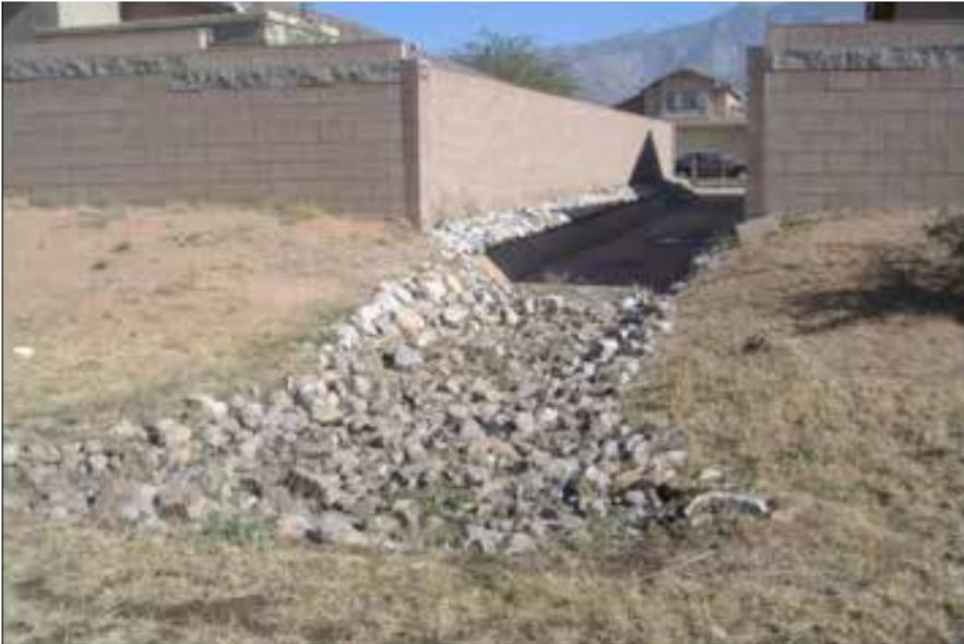
**A basin inlet and concrete drainage channel that are in design condition.**
