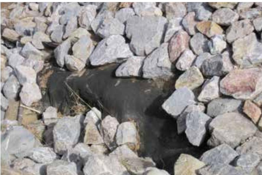
**Riprap erosion protection that has shifted over time, exposing the underlying filter fabric.**
