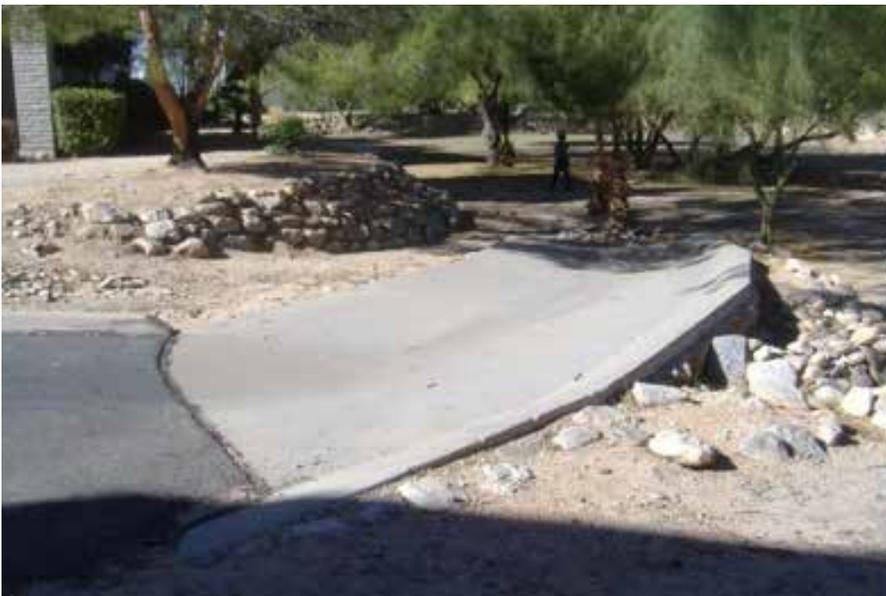
**A drainage easement with concrete apron for street flow.**
