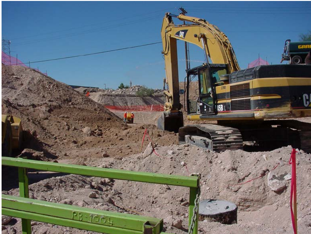
Photo 1 - Cherry Fields construction
