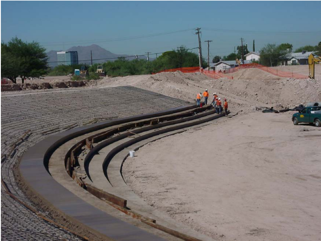
Photo 3 - Cherry Fields construction
