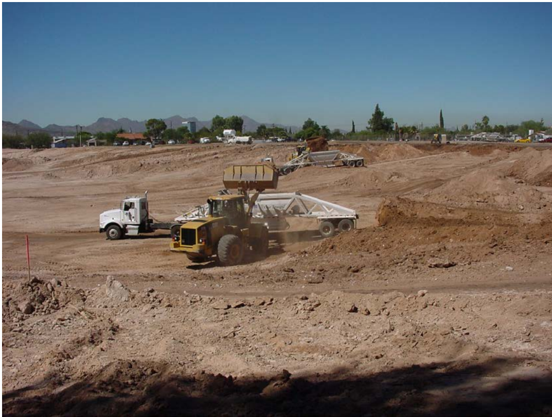
Photo 4 - Cherry Fields construction
