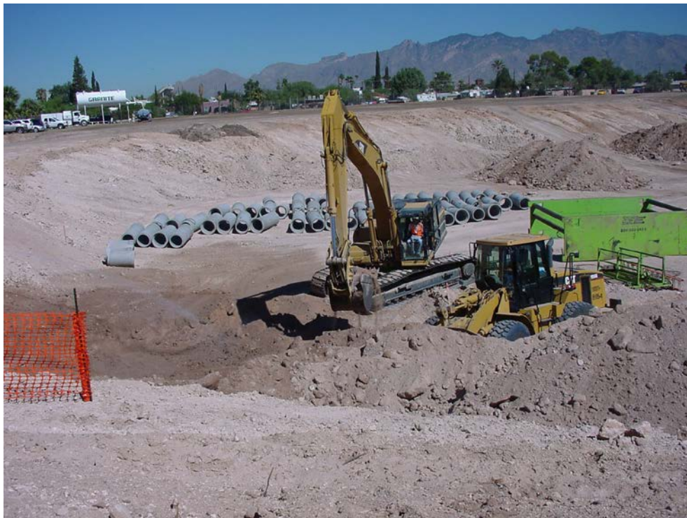
Photo 2 - Cherry Fields construction
