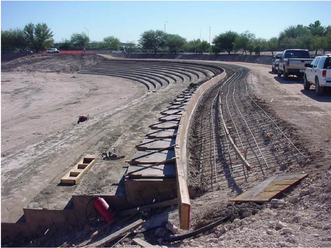
Photo 5 – Cherry Fields construction
