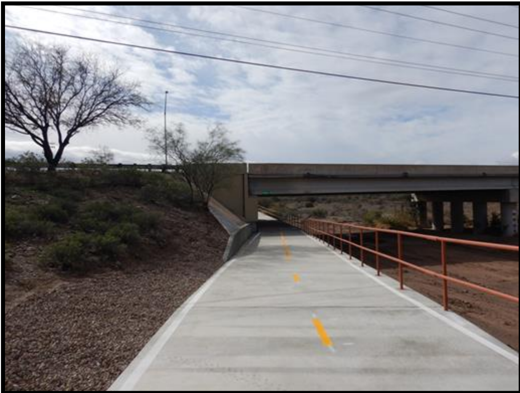
Modified Underpass: Pathway width = 12 feet, Bridge clearance height = 10 feet
