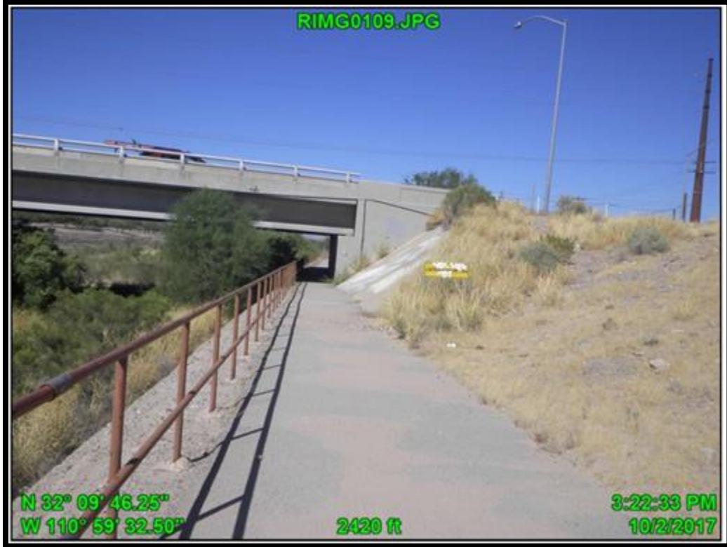
Original Underpass: Pathway width = 6 feet, Bridge clearance height = 8 feet
