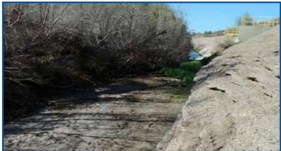
Below: Outfall area after the clean-up.
